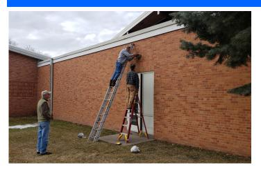
Trustees Steve Knopp, Harvey Erstad and Tom Wellman replaced all of the light bulbs around The PORT with LED lights. They also replaced the ballasts in the light fixtures. Next, new lights will also be installed on our sign in front of the church.
